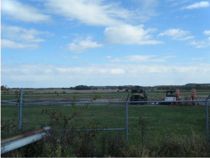
Figure 6. Existing types of fence surrounding the AOA.
