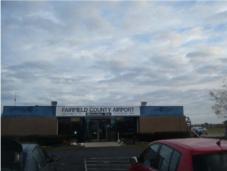
FP 1: Looking north.
